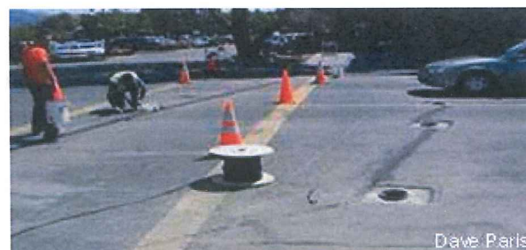
In-pavement flashers at crosswalks are also an option that can be considered.
