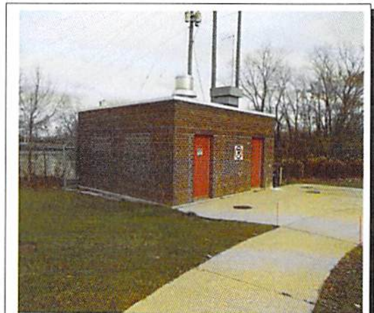
Figure 1 Existing South 19th Street Pumping Station
