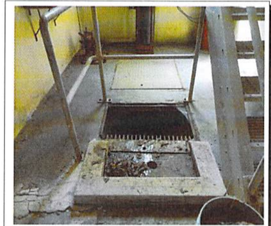
Figure 3 Existing Bar Screen in the Wet Well Area
