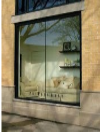
Figure B2.2: Clear glass allows visual access to the retail storefront display.
