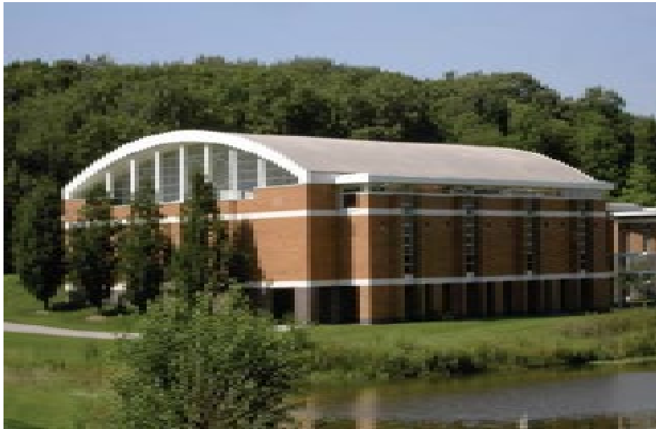
Figure C2.3: Effective use of modulation and horizontal articulation to minimize the appearance of bulk.
