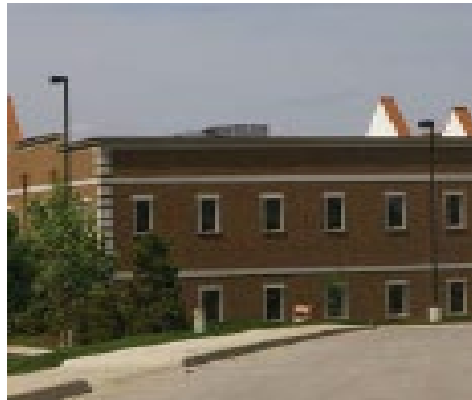
Figure C4.2a: AVOID extending vertical façade of a building face above the actual parapet or roofline to give the appearance of a false front. AVOID unscreened rooftop mechanical units.
