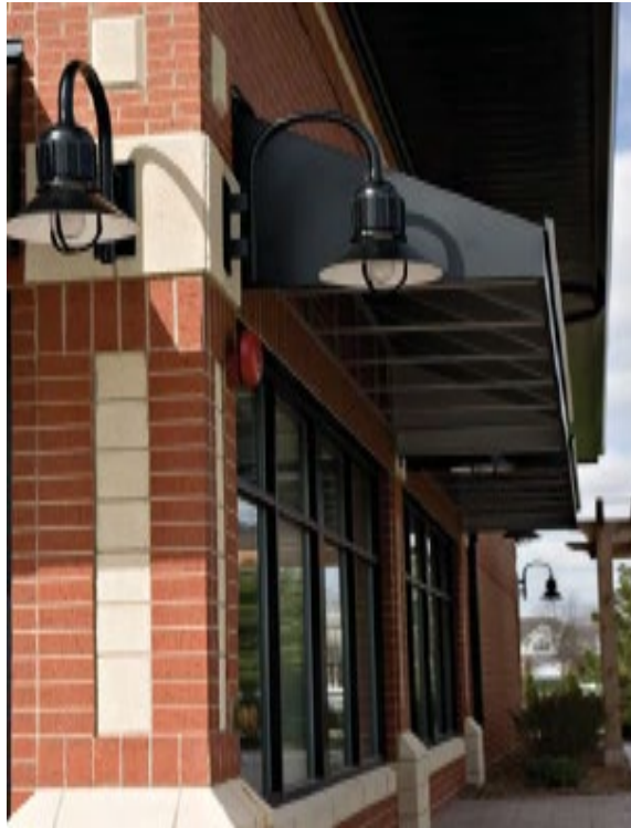
Figure B5.4: Patterned masonry detail and light fixtures enhance pedestrian character.
