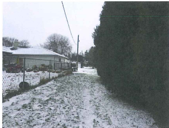
Looking west on existing sewer easement, towards Lawton Terrace. Site constraints will make open-cut sewer installation challenging, even with additional easement acquisition.
