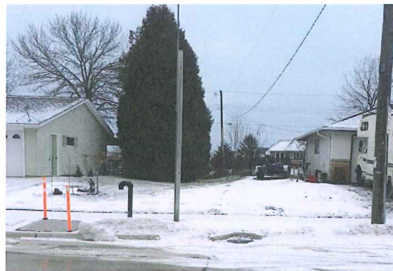
Looking east, view of existing Lawton Terrace lift station and sanitary sewer easement.
