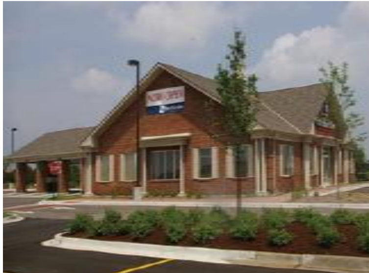
Figure C7.3: Secondary façade enhanced by use of varied rooflines, architectural detail that is consistent with front façade.
