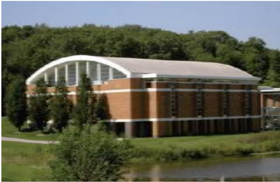
Figure C2.3: Effective use of modulation and horizontal articulation to minimize the appearance of bulk.
