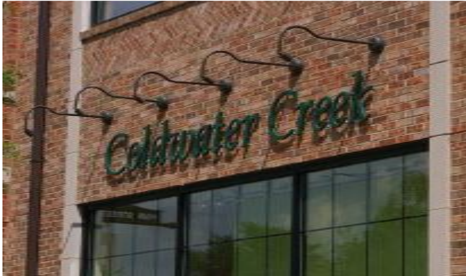
Figure C9.4: Pedestrian-oriented building signage with exterior mounted lighting.
