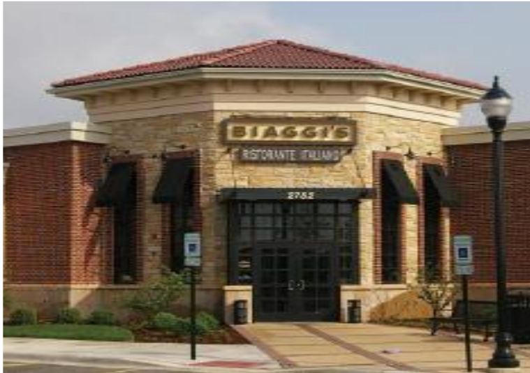
Figure B5.1 and 5.2: This building incorporates masonry knee wall and decorative cornice elements.
