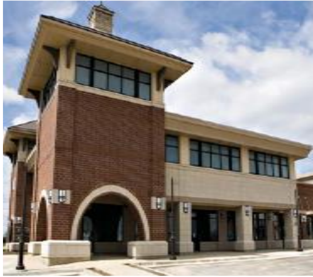
Figure C1.2b: Balance is created by tower on the left side offsetting the longer section to the right.
