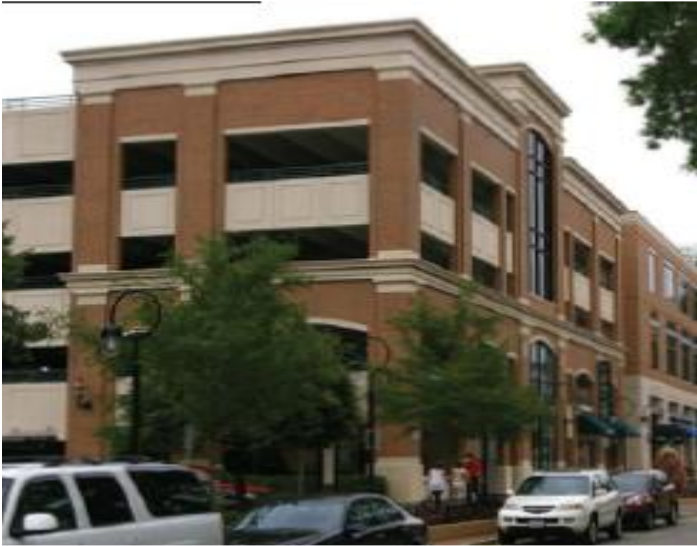
Figure C2.1a: Vertical brick articulation combines with horizontal stone/ precast concrete banding to form overall grid frameworks. Cornices unify the top of the building.
