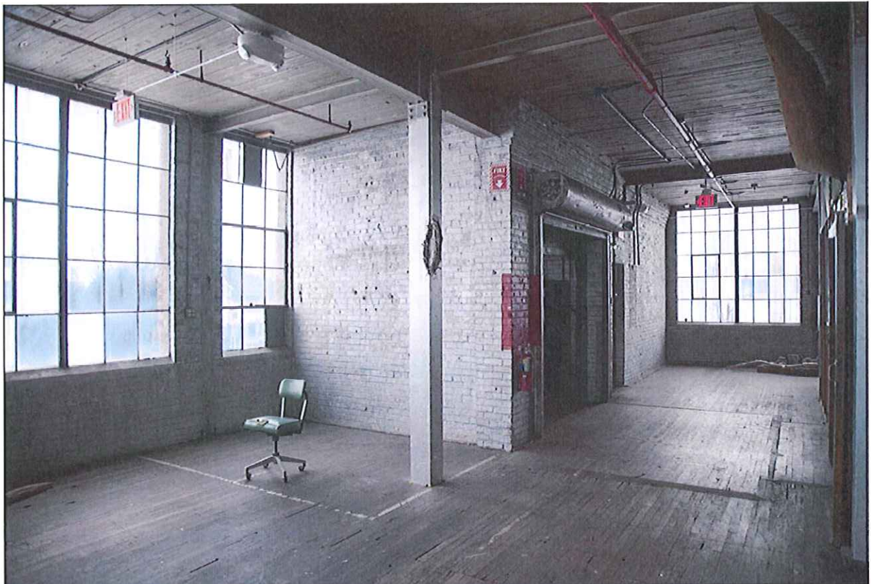
Image 29: Typical floor, view looking northwest
