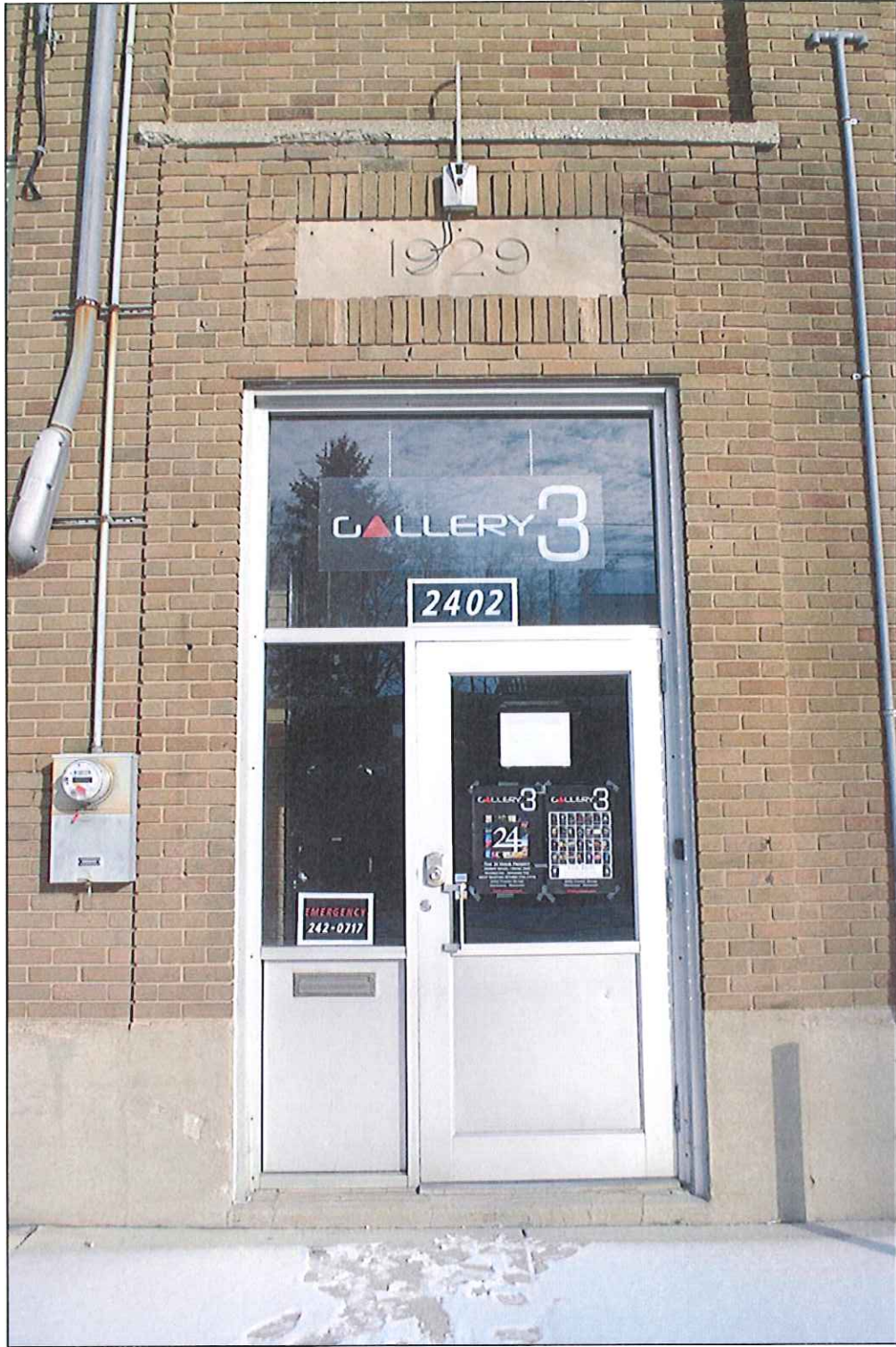
Image 21: Mirro Plant #3 in 2013, south entrance view looking north.
