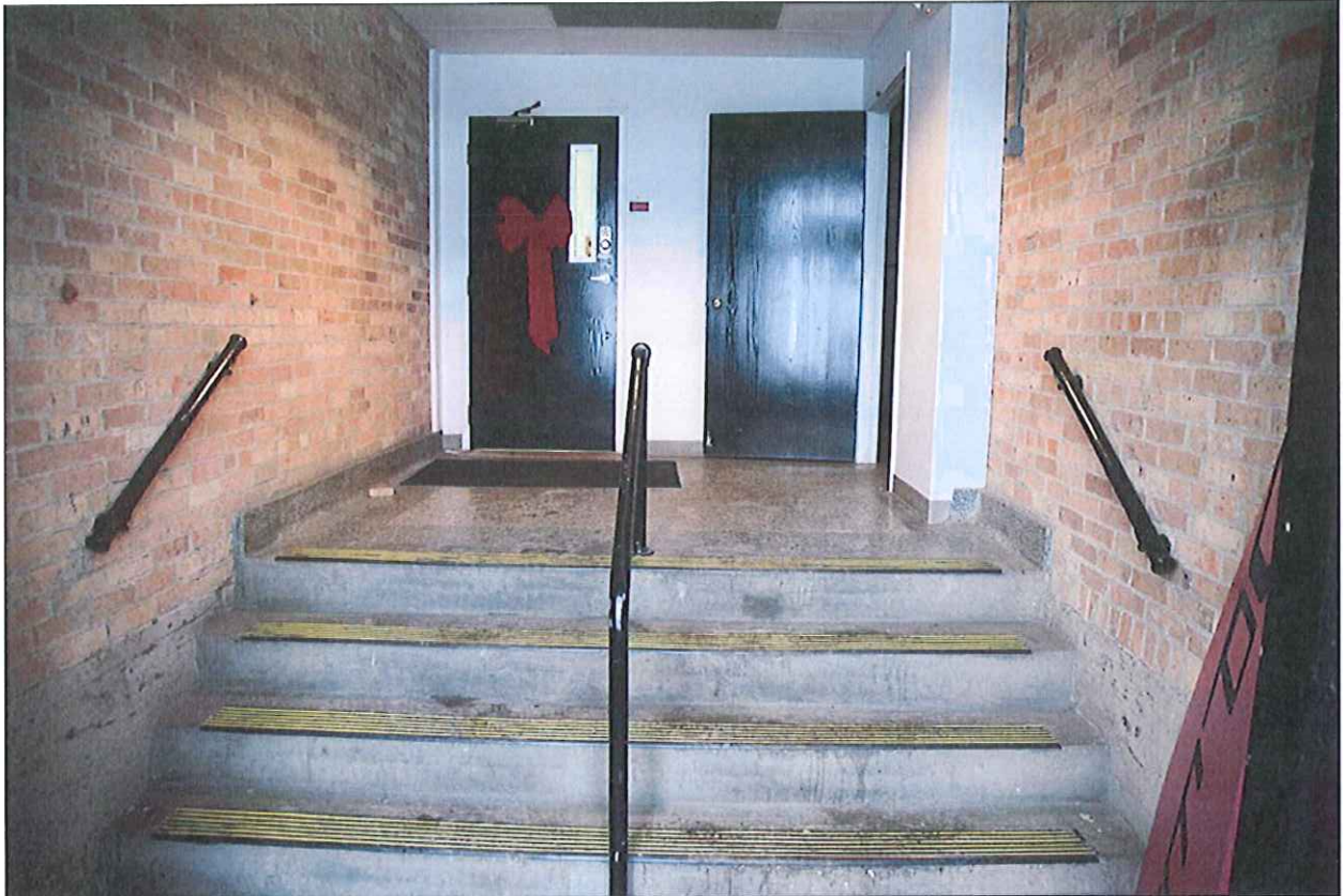
Image 24: First floor vestibule, view looking north
