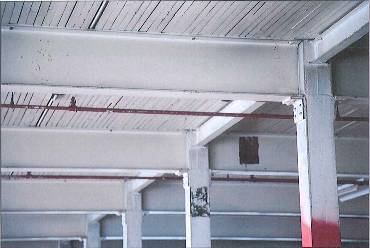
Image 30: Typical floor, detail of exposed structure.
