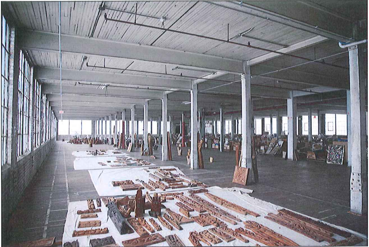
Image 28: Typical floor, view looking west.
