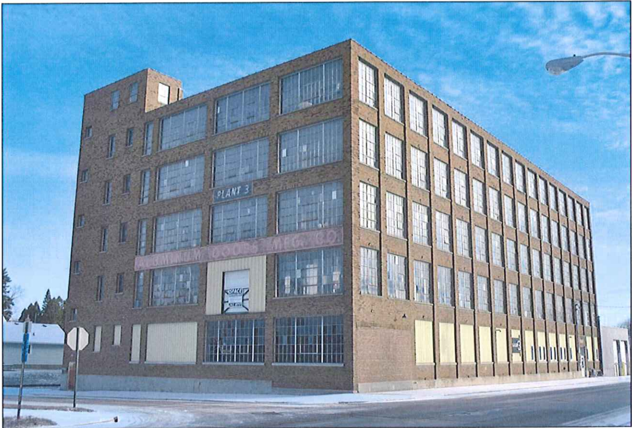
Image 19: Mirro Plant #3 in 2013, south and west elevation view looking northeast.
