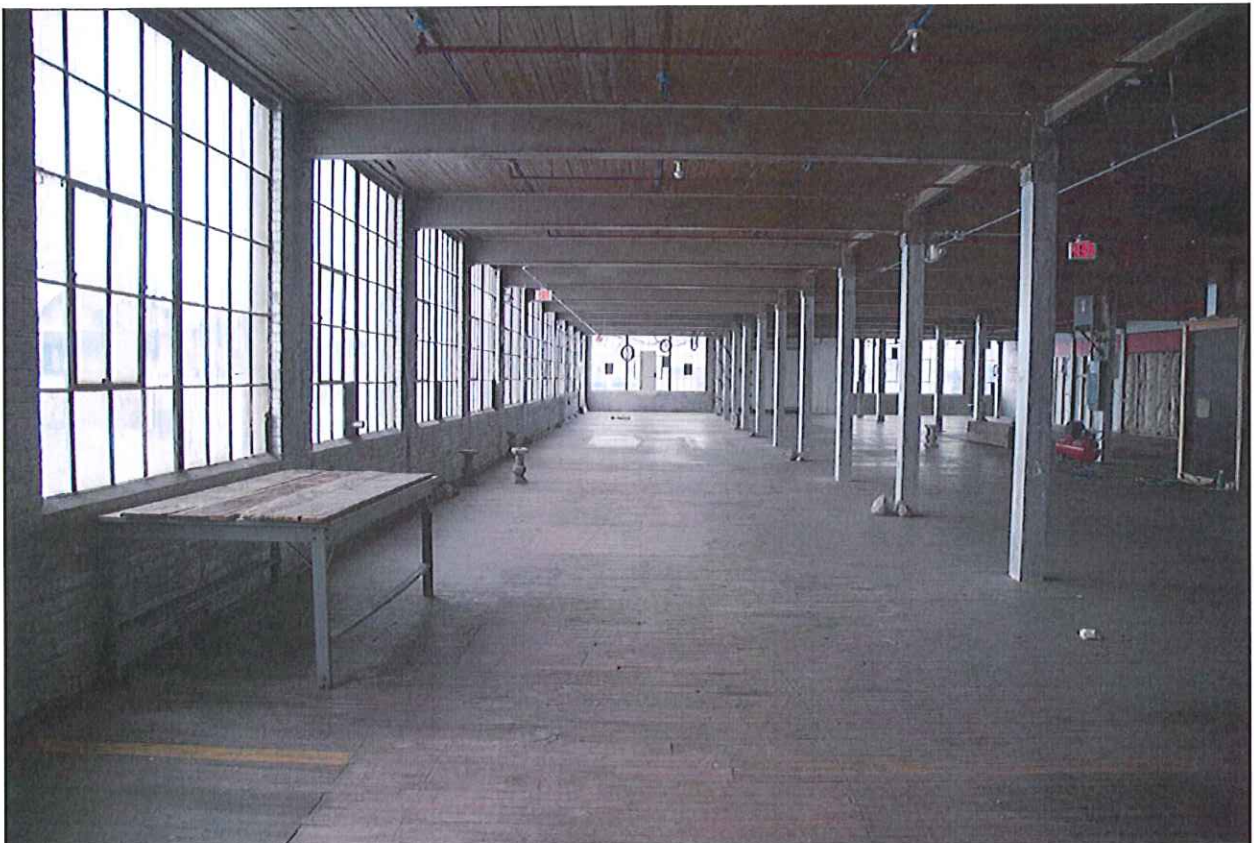
Image 25: Typical floor, view looking west.
