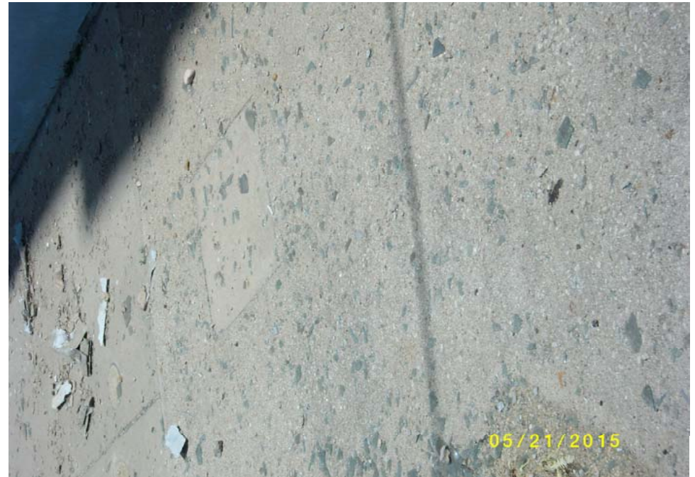
Broken glass accumulating on sidewalk.
