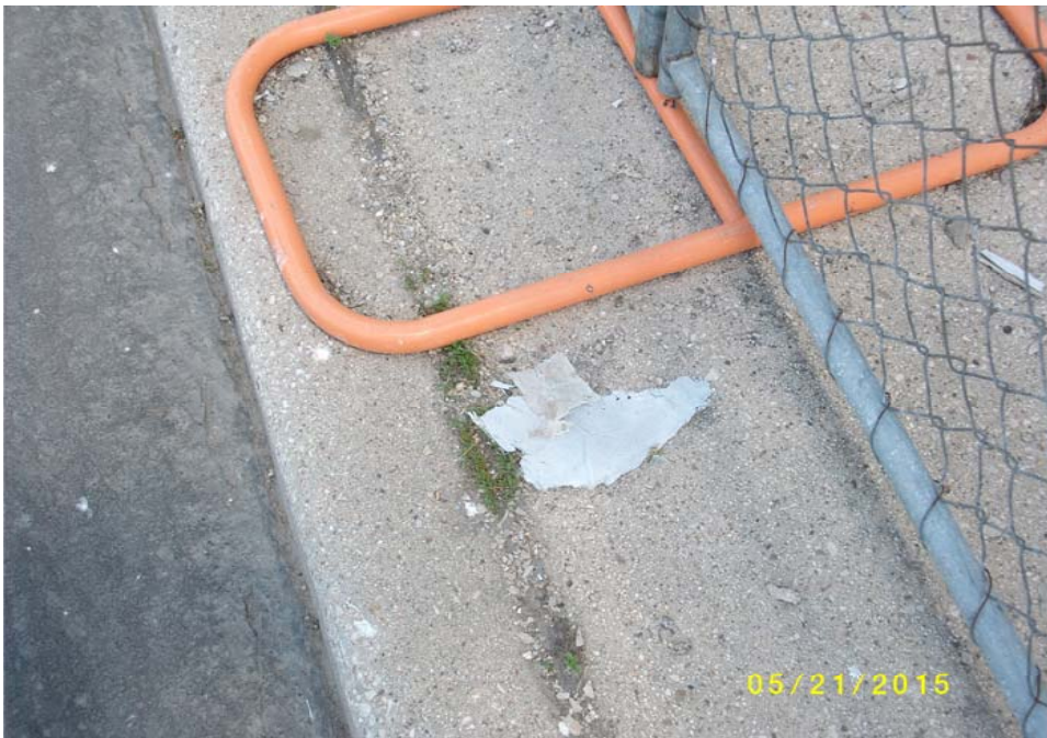
Asbestos containing material on sidewalk outside of construction fence.
