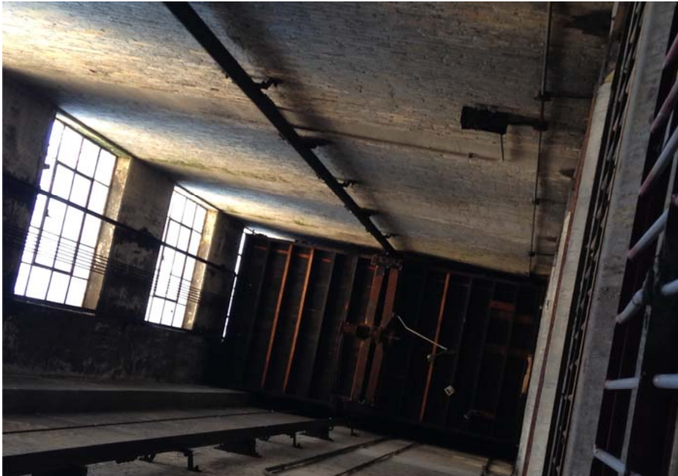
Open elevator shaft.
