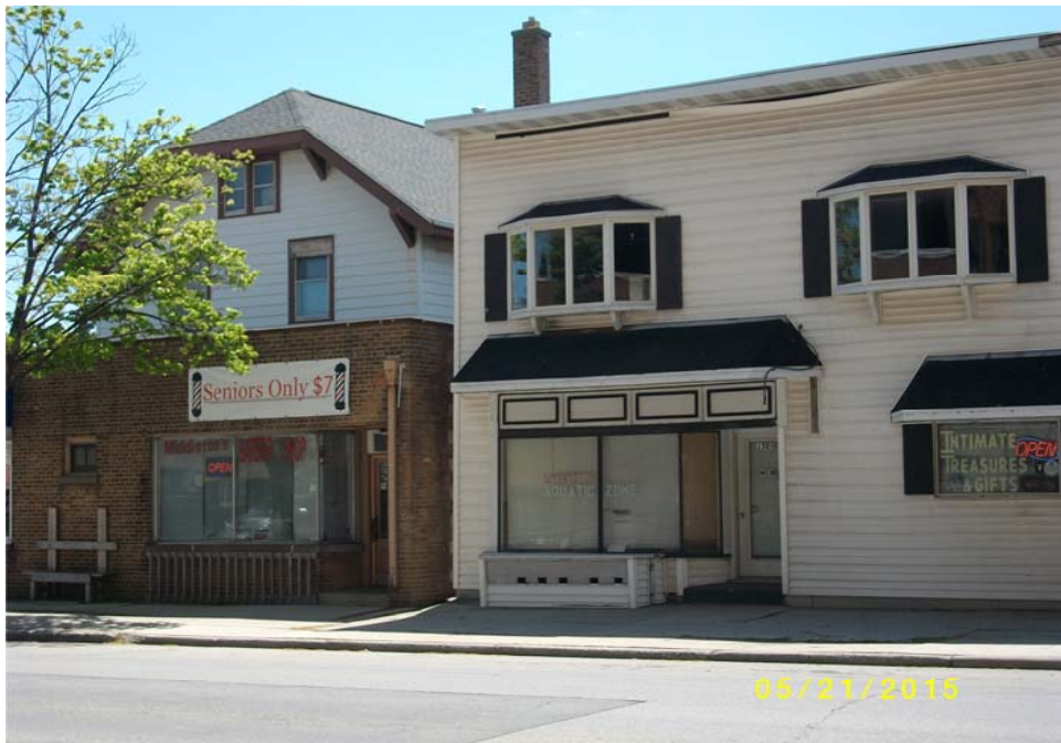
Properties in surrounding blocks; deteriorated conditions.
