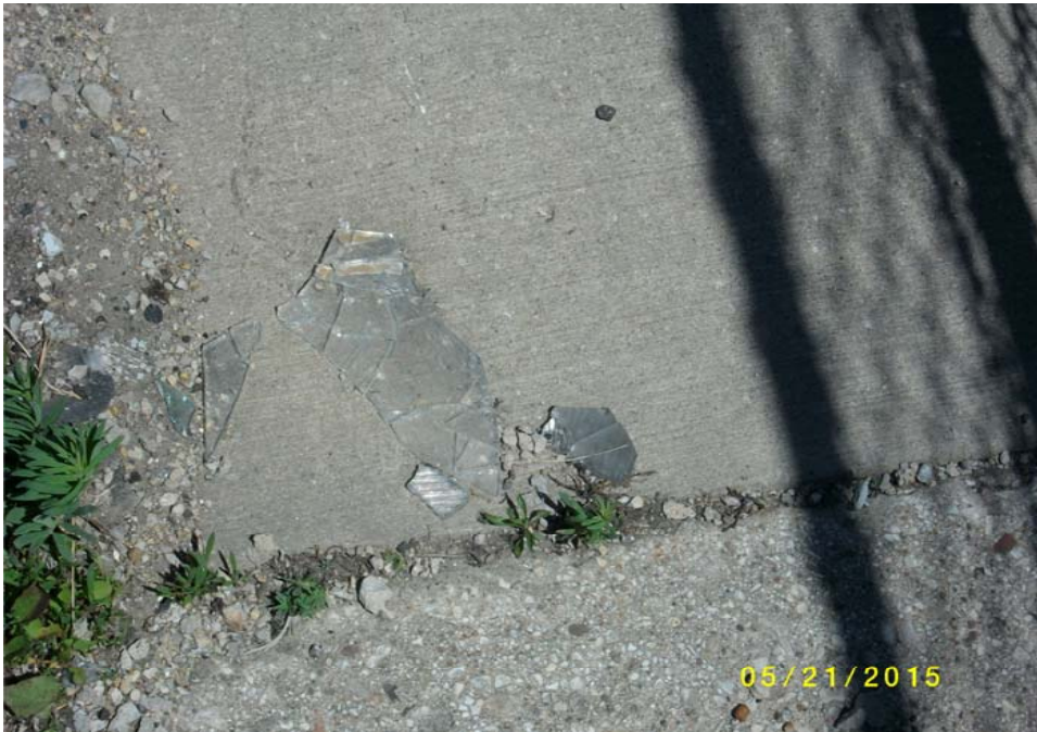
Broken glass on sidewalk outside of construction fence.
