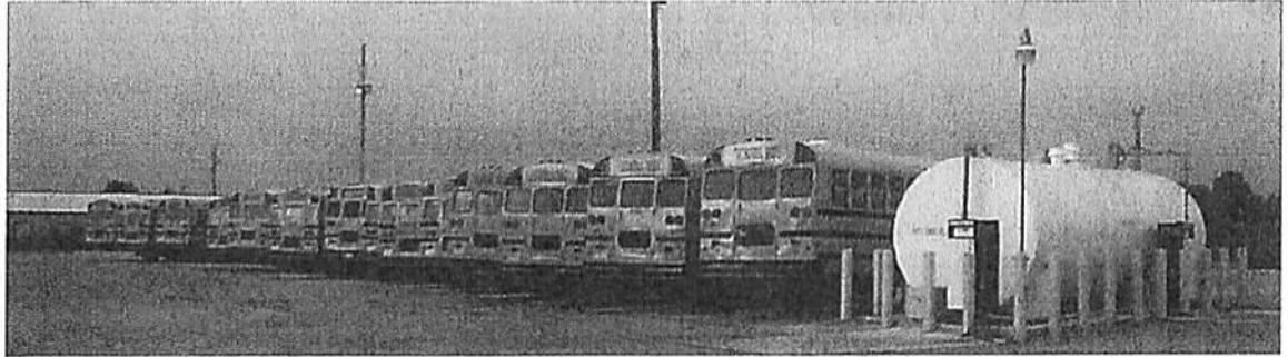
A view of the 10,000-gallon fuel tank. Also, a view of part of the bus fleet that could be used as spares if needed.
