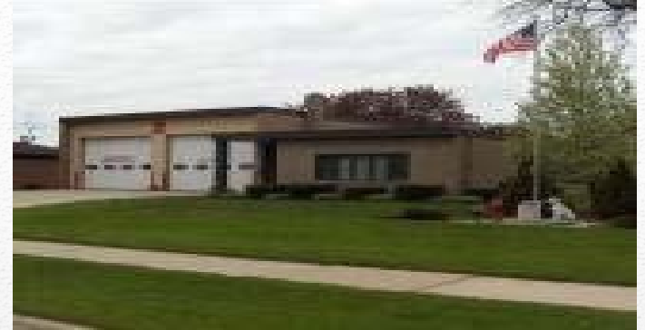
Station 2: 1410 N 8 th St. Built 1957
