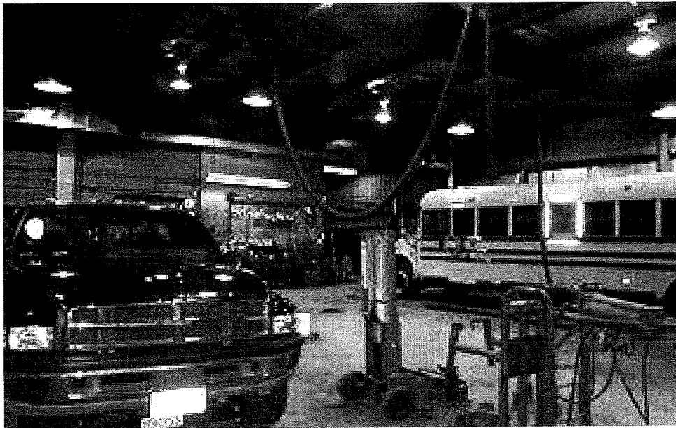
A view inside the three-bay maintenance area.
