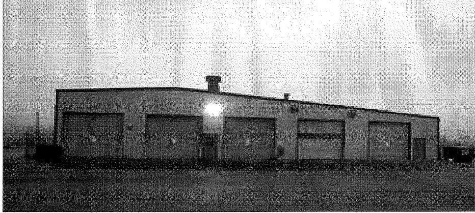
Back of Brandt Buses building (where Assist-To-Transport, LLC has its office) showing the three-bay maintenance stalls on the left. The white door represents our bus wash stall. The door on the far right is a storage and additional maintenance stall.
