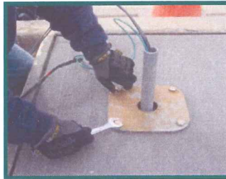
Finished Concrete Pad
