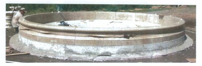
Now that each section is sitting on epoxy, the surround must be pulled tight for correct alignment. We suggest using a simple ratchet strap to pull the sections in place and make final adjustments.
