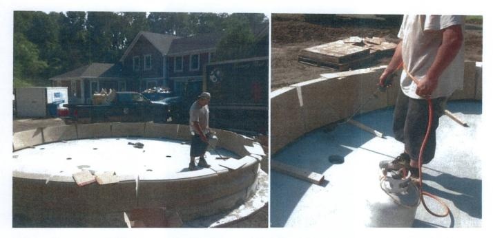
While holding the cardboard between the sections, carefully tilt the sections back to remove the wood blocks and set back on the concrete.
