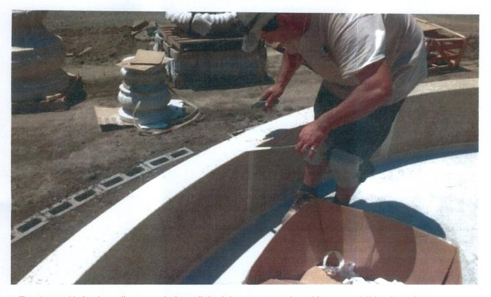
• Touch up with fresh caulk as needed so all the joints are smooth and have no visible air pockets.
