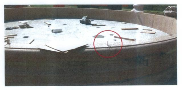
• Use 1/4" shim shingles pushed in from the top down to maintain spacing.
