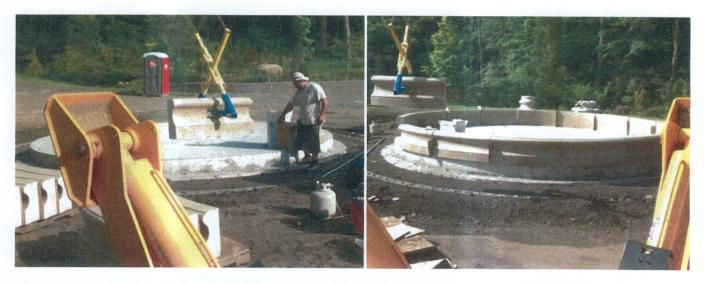
• Dry-set all sections in their correct locations and make any necessary adjustments at this time.
