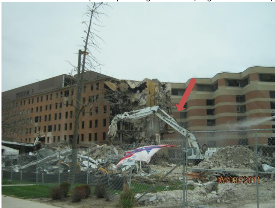
3. Concrete multiple story building demolition (long reach excavator)
