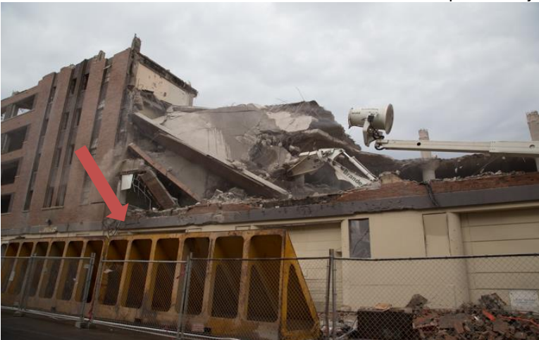
6. Debris Shields to protect adjacent structures and property.
