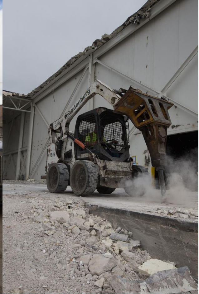
8. Skid steer with hydraulic breaker (jack)
