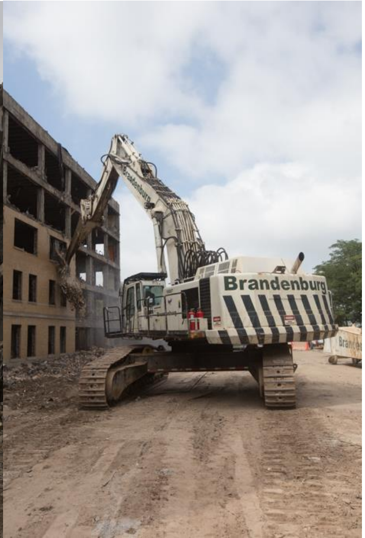
3. Concrete multiple story building demolition (long reach excavator)
