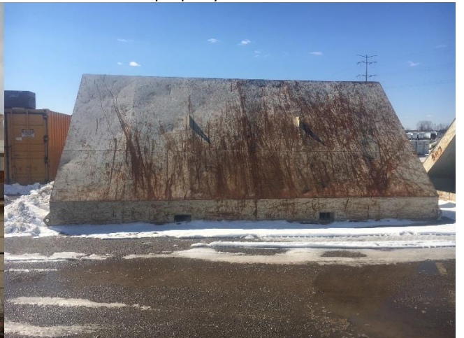
6. Debris Shields to protect adjacent structures and property.
