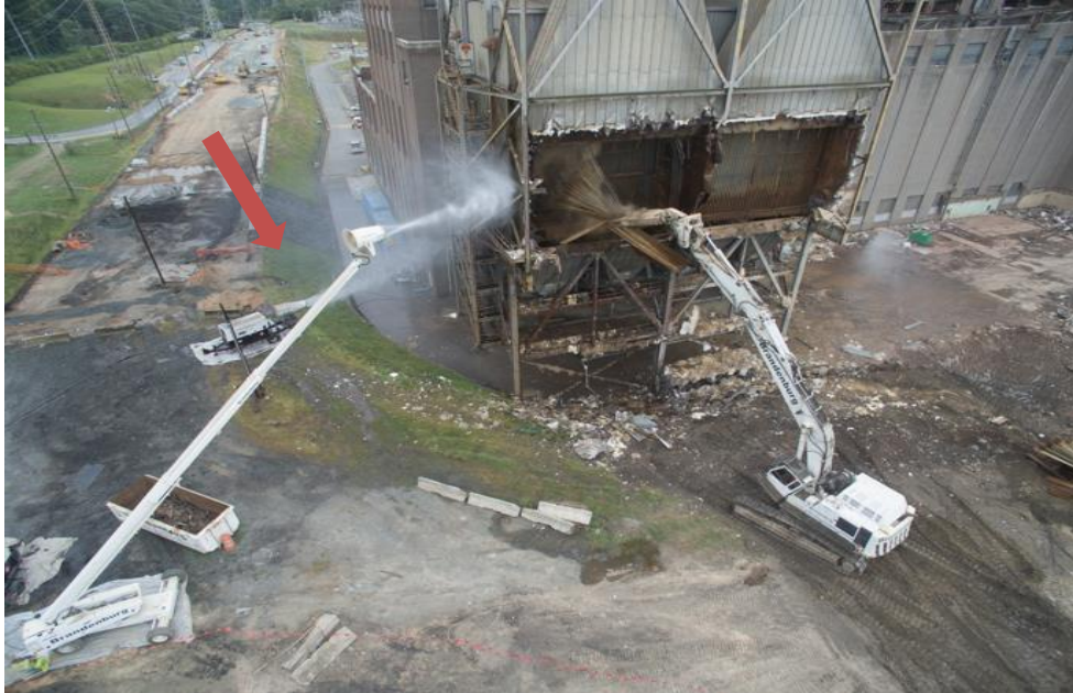
5. Aerial and ground dust suppression
