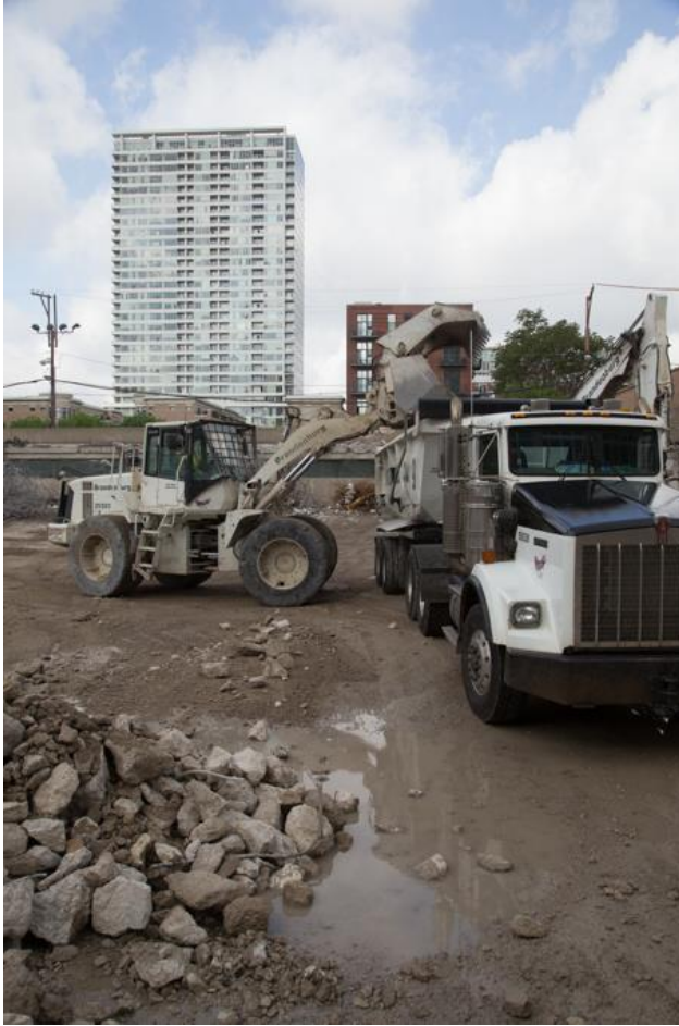
7. Loading trucks with demolition debris
