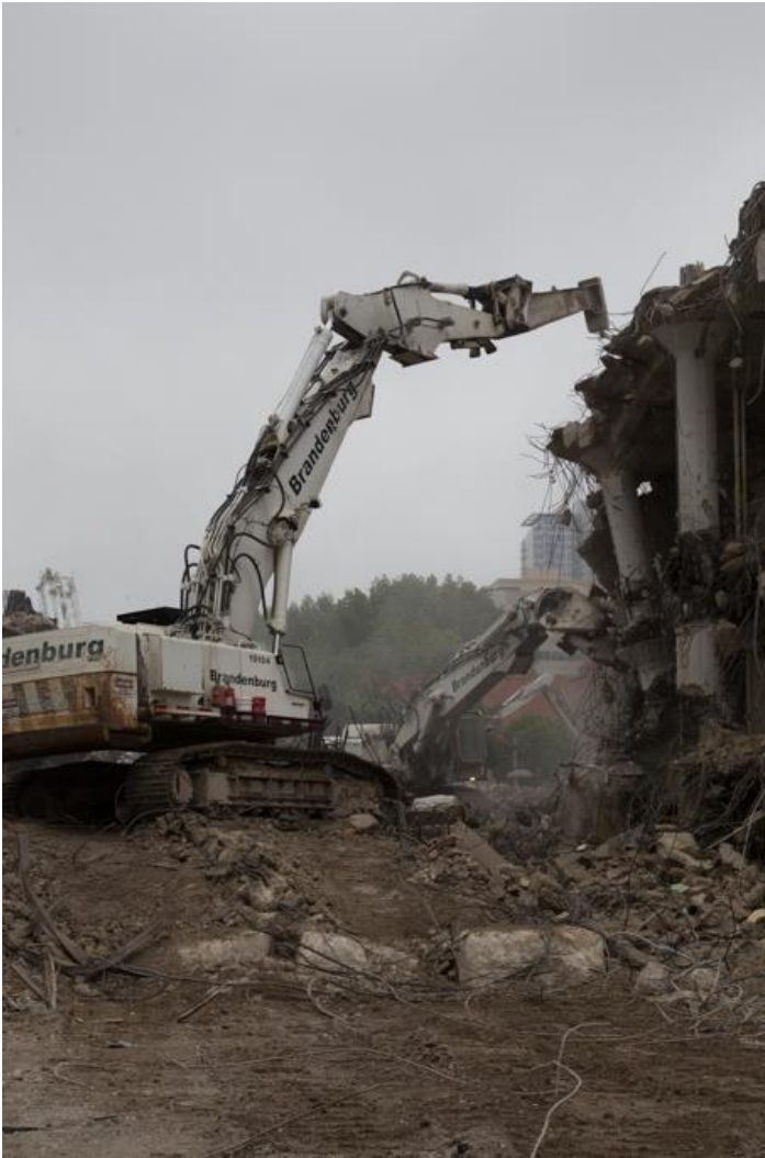
3. Concrete multiple story building demolition (long reach excavator)
