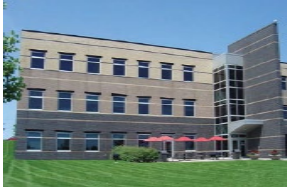
Figure B3.2: Entry is clearly marked by a tower feature, variation in color and material, canopy, and recess/projection.
