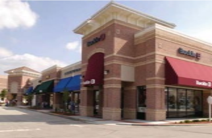
Figure C2.2: Combined vertical articulation and modulation minimize the appearance of a long, massive wall.
