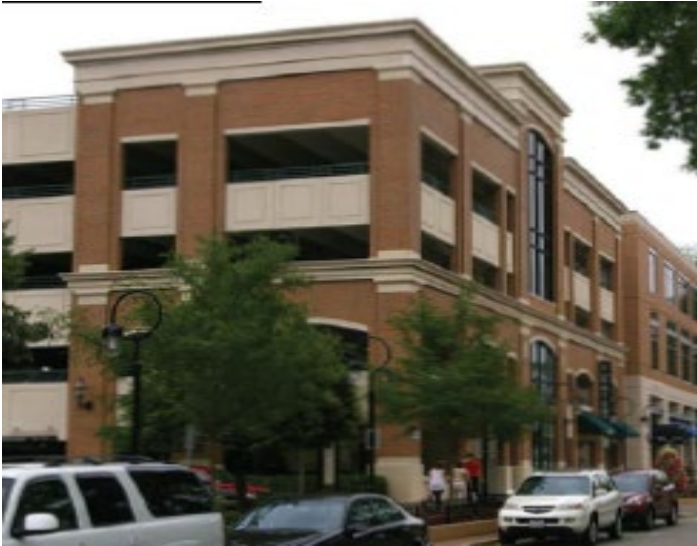
Figure C2.1a: Vertical brick articulation combines with horizontal stone/ precast concrete banding to form overall grid frameworks. Cornices unify the top of the building.
