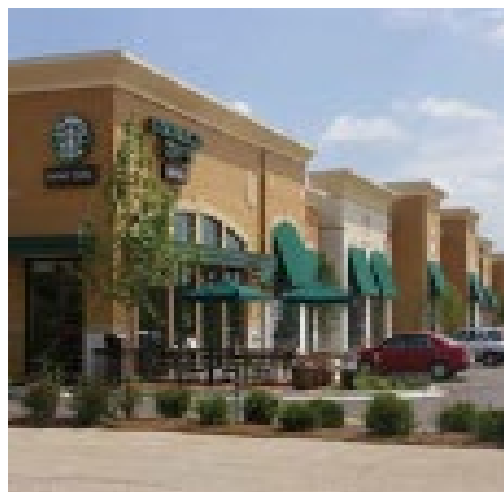
Figure C4.2b: Raised parapet with substantial depth creates varied rooflines. Rooftop mechanicals are completely screened by the parapet.
