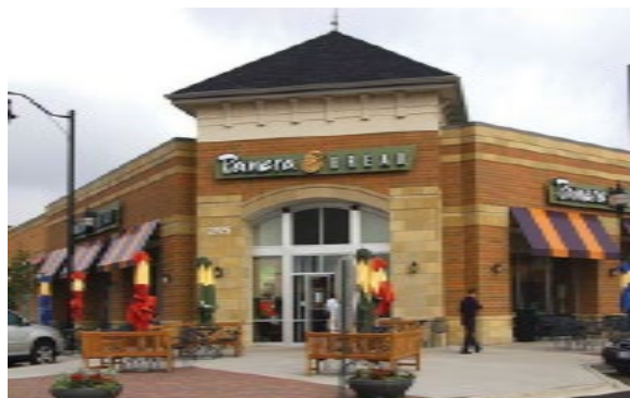
Figure B3.3: Arched entry with pedestrian lighting transitions the overall building to pedestrian scale.
