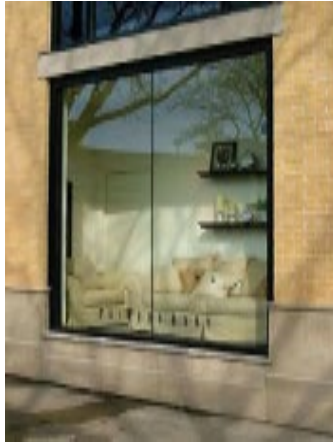
Figure B2.2: Clear glass allows visual access to the retail storefront display.
