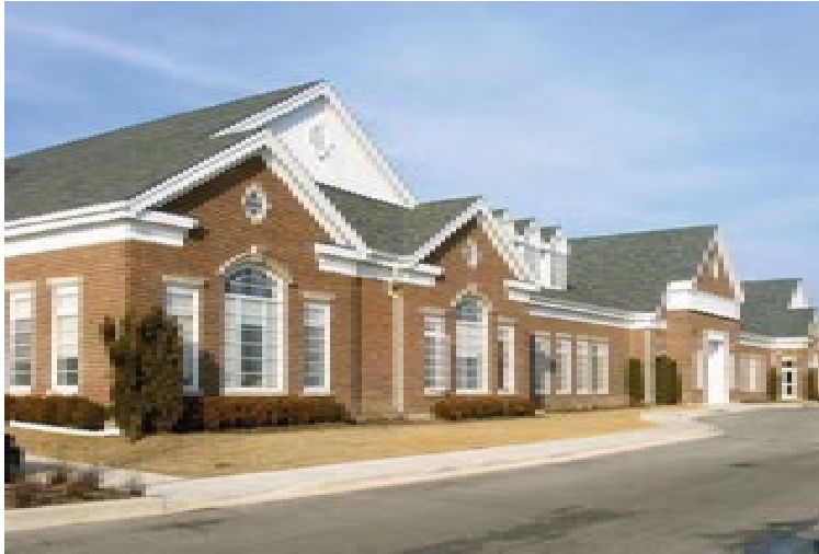
Figure A2.2b: This building uses varied roof forms and façade planes to reduce apparent size.
