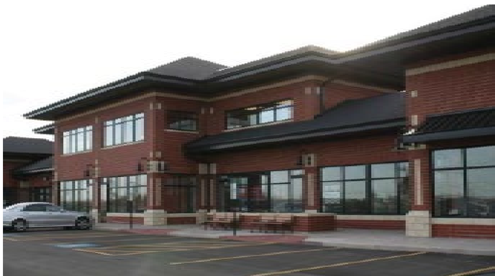
Figure C1.1a: Building materials and massing unify the structure as a whole.
