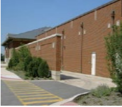
Figure C8.2b: Effective use of a screen wall to conceal loading functions.
