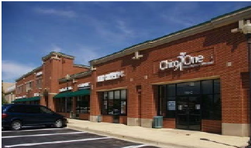
Figure C9.1a: Scale of signage is appropriate for building. Multiple signs are displayed in a consistent manner.
