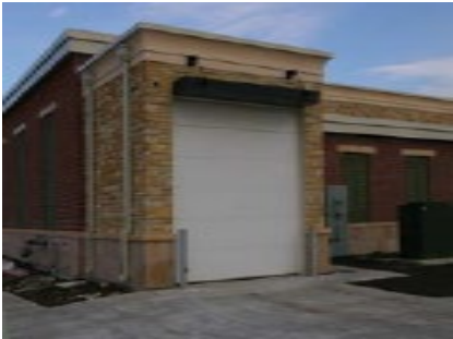
Figure C8.2a: Internal loading area.
