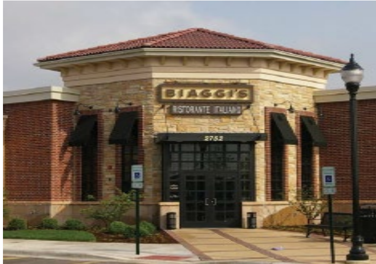
Figure B5.1 and 5.2: This building incorporates masonry knee wall and decorative cornice elements.
