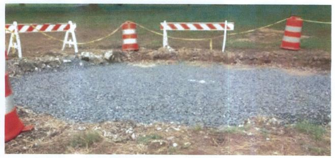
A well-compacted base is required for the fountain slab. Depending on soil-type, or if fill is needed to compensate for uneven terrain, crushed stone is a good choice for base. Crushed stone will also aid in drainage.
