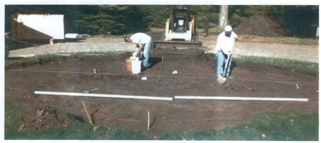
· Locate and mark the center point of the fountain as all measurements will be based off the center point.
