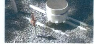
· Compact the soil/gravel around the pipes where trenches were made.
