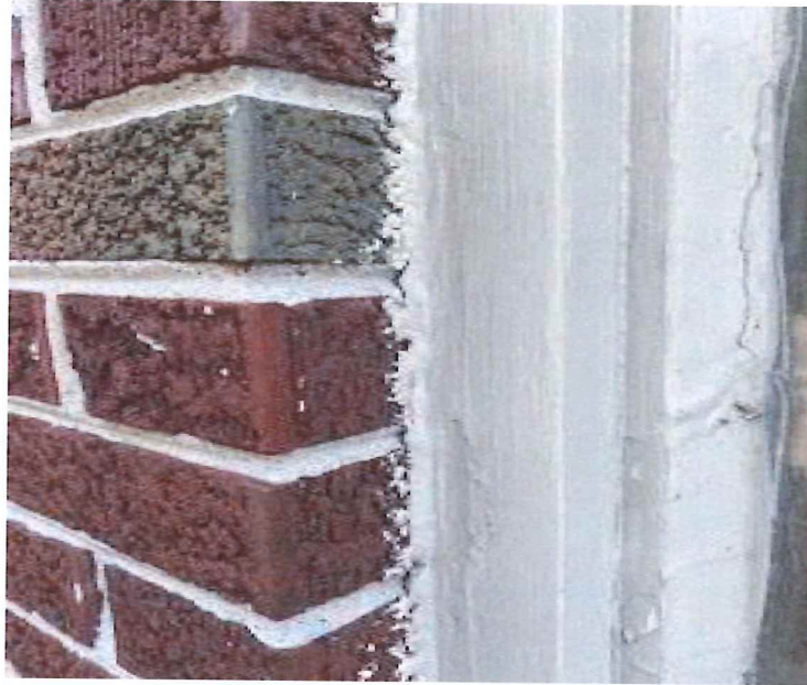
Photograph 15 – A view of the caulking and window glazing.
