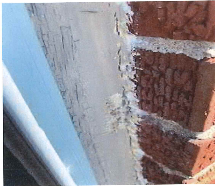
Photograph 14 – A view of the beige/gray window caulking.
